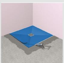
G When the screed is set, remove rubber protection strip and fill the gap with Mega Power Sealant, as well as gaps between the shower base and the walls. If tiling over Kaskade, prime the surrounding concrete before tiling with two coats of SBR Tilers Primer, diluted 3:1, to fully waterproof it.
